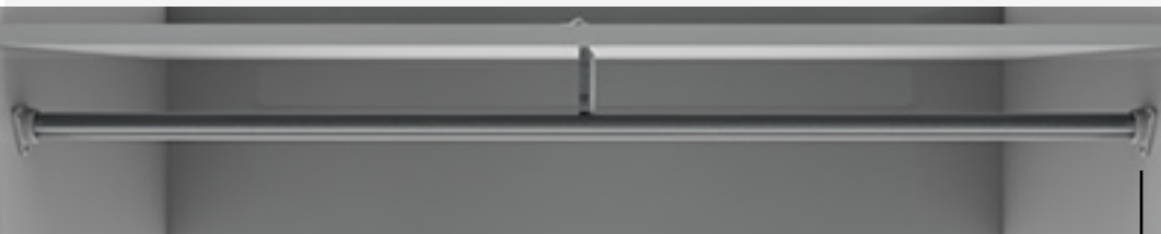
Wall to wall closet led rod (Alu-Round) installation
